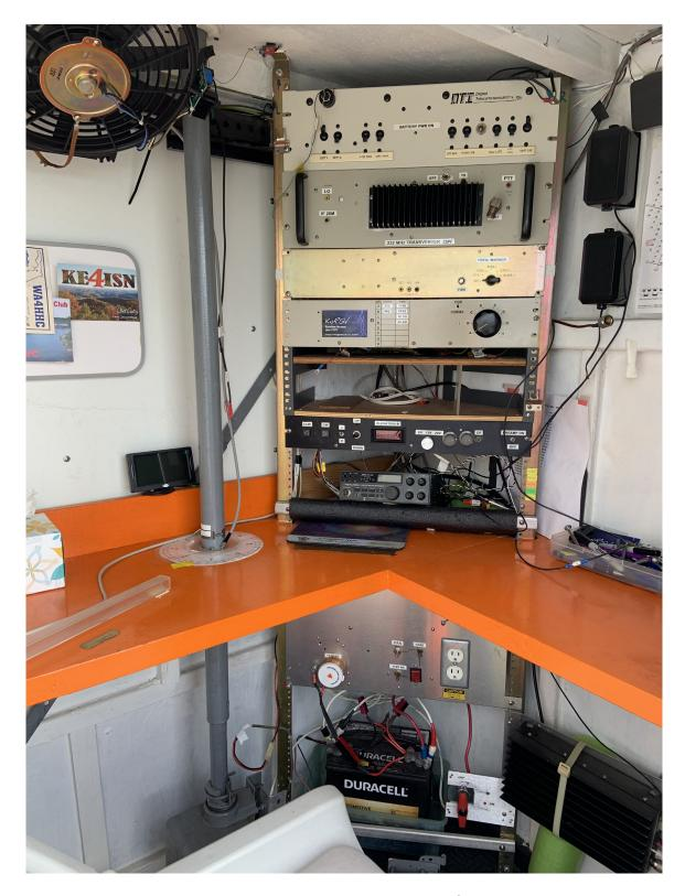
The compact trailer has the antenna mast resting on the floor inside the trailer, and going through the operating table with a compass taped to the table surface.
